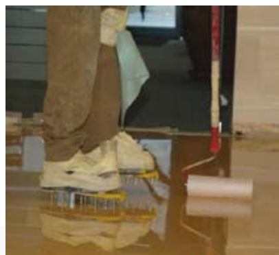
Tamafloor Coating Application
